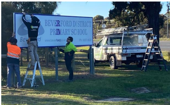
Erection of the new sign on the highway
